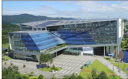
Pan-gyo Center in Seoul Metropolitan area (2015.12)
